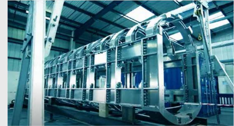
Leading design of the award-winning King's Scholars Pond sewer project (UK) to **rehabilitate a Victorian-era underground structure**, extending the life of the pipe bridge by 120 years. The team's clever solution involved strengthening the sewer from the inside, eliminating a potential three-month road and rail closure to one of the busiest intersections in London and **saving ~26,400 tCO<sub>2</sub>e**.
